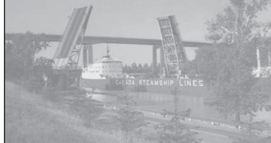
Homer Bridge • Welland Canal, St. Catharines, Ontario, Canada
